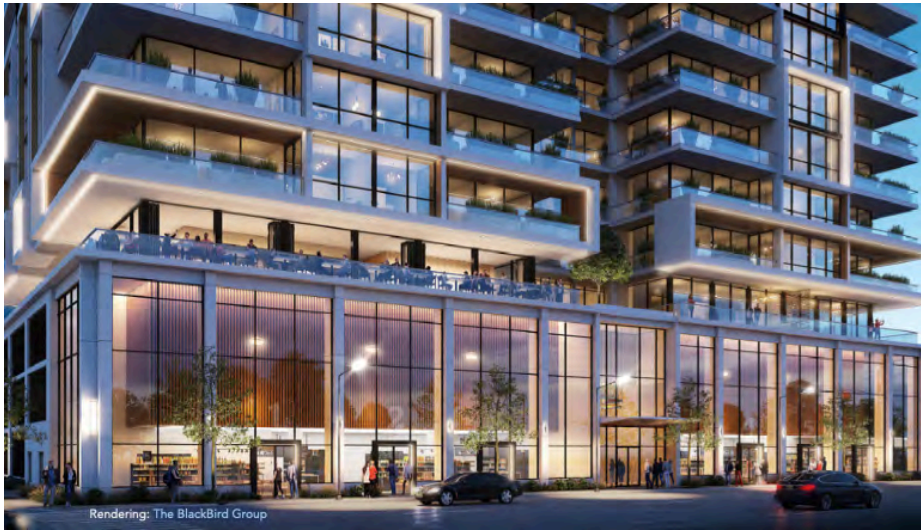
Renderings and plans for the former 'steel structure' redevelopment effort, Seaside Heights, N.J. (Source: SSH Redevelopment Plan Deck)
